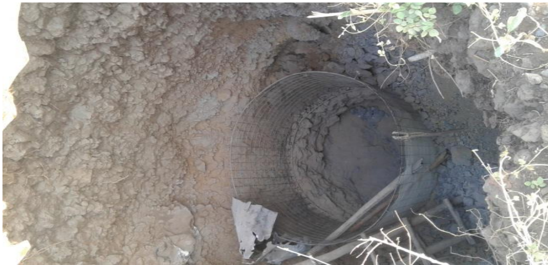
Figure (i) An abandoned pit which was being dug as a shallow water well
