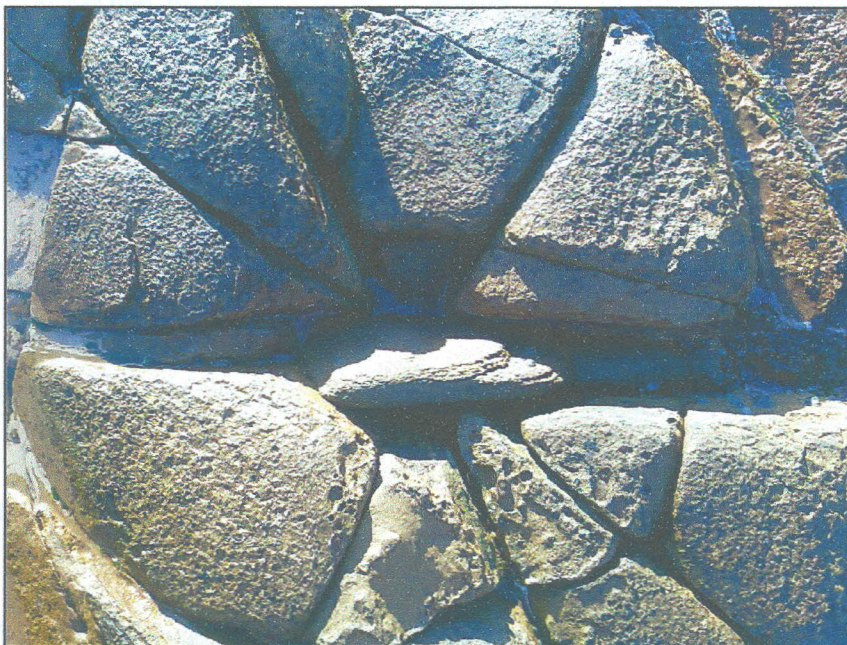
Fig 3-3; Fracturing in rocks (Gregory, 2006)
