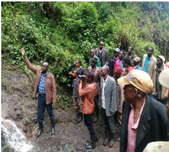
Plate 2: Very steep Kapkese slope where landslide occurred in December 2015
