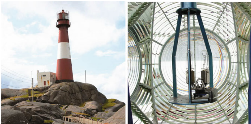
Fig. 11.24 Eigerøy Lighthouse is a powerful monument from a time before the GPS made its entry. To the right: the lens system that surrounds the light bulb is impressive. There are three equivalent lens systems that are located 90^\circ apart. The last “wall” is open to permit entry. The lens systems are over two metres tall
